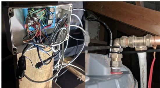
Fig. 3: The control box appears on the left-hand side; a representative flow sensor (F1, hot water outlet) is shown on the right hand side.
